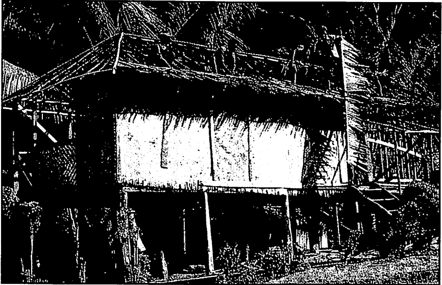
A house being roofed with palm thatch. The leaves are boned then folded over a stick and stitched on. It is amazingly rain-proof.
