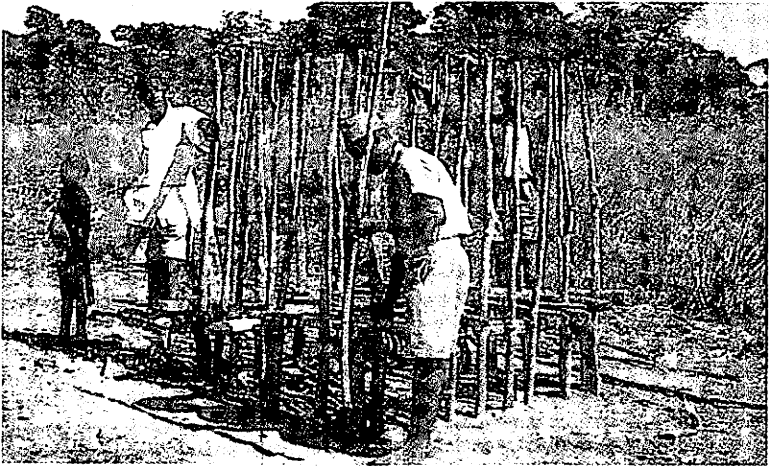
Building a grain storage house.
