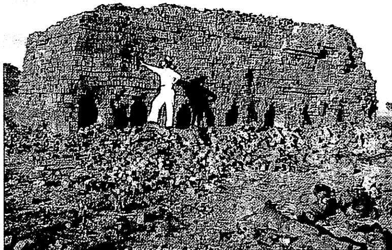
Alvin standing near a kiln of bricks which have been burned and are now ready for use.
