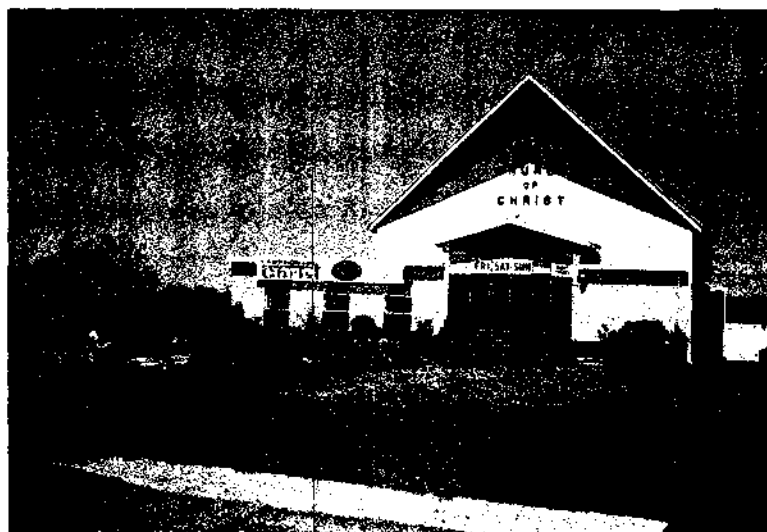
After remodeling was finished.
