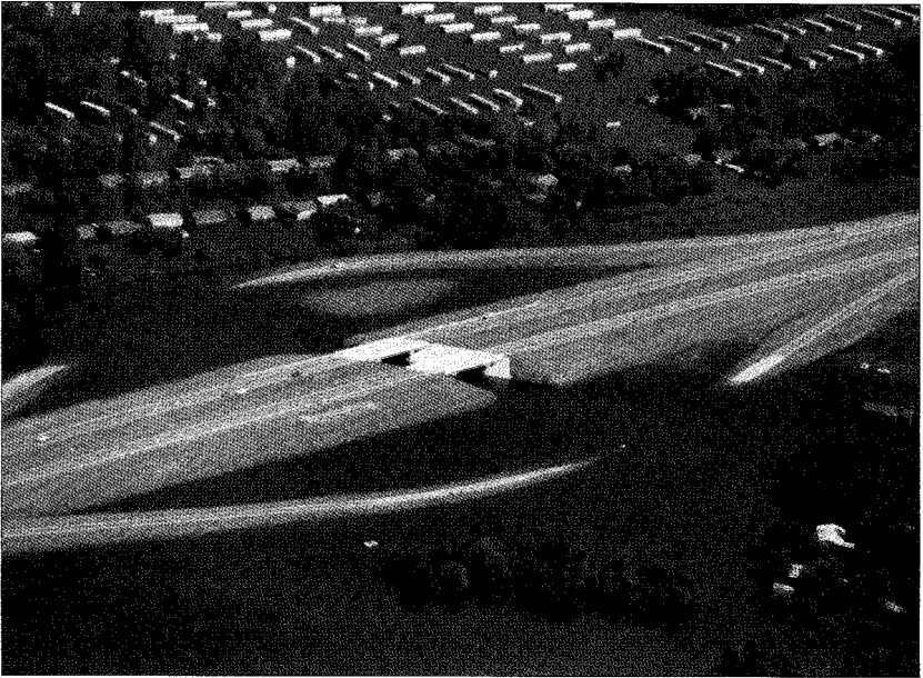
An aerial view of Interstate 40 and surrounding houses in the tragic flooding in North Carolina in 1999.
