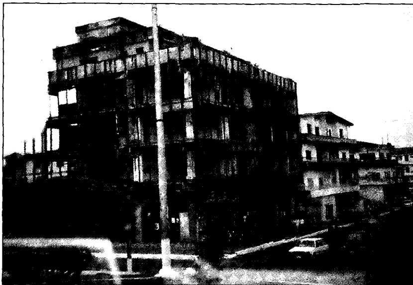
The skeletal remains of a multi-storeyed building in Monrovia — typical of so many homes and businesses throughout the country.
