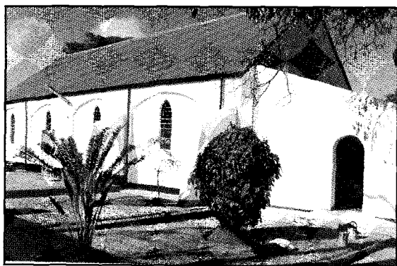
Mutare church building.
