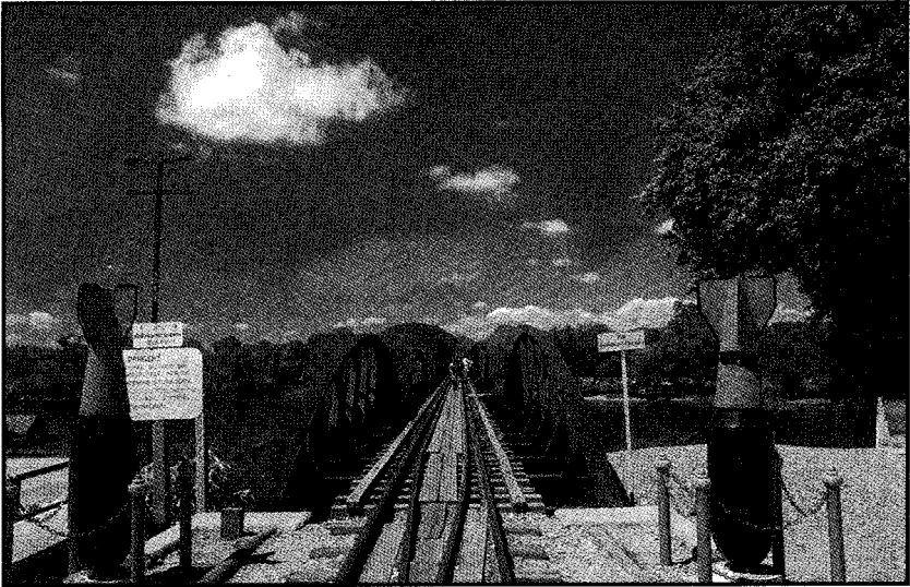
The famous “Bridge over the River Kwai” built by Allied prisoners under Japanese occupation during World War II.
