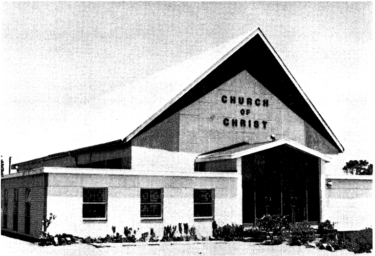
21. Pickering Street building in Port Elizabeth, after remodeling.
